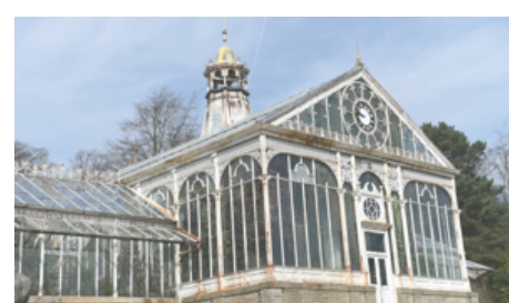
Work begins to protect Corporation Park conservatory December 8, 2023 in "Blackburn"
